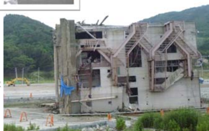
Architectural remain of Tsunami
